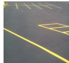
**Sealed and Striped** is the finished asphalt. The real benefit to sealing is the protection it provides to the asphalt surface. It also doubles the service life of the pavement.
