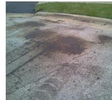
**Petroleum Spills** of Gasoline, oils, and jet fuels dissolve asphalt causing it to soften and eventually deteriorate.
