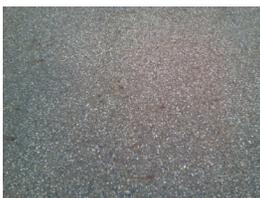
begins to oxidize and weather soon after installation. Moisture penetrates the asphalt causing further damage and deterioration to the pavement.
